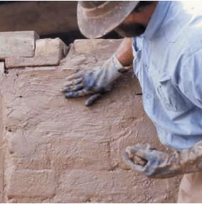
REN - Render Earth render system, using local materials
