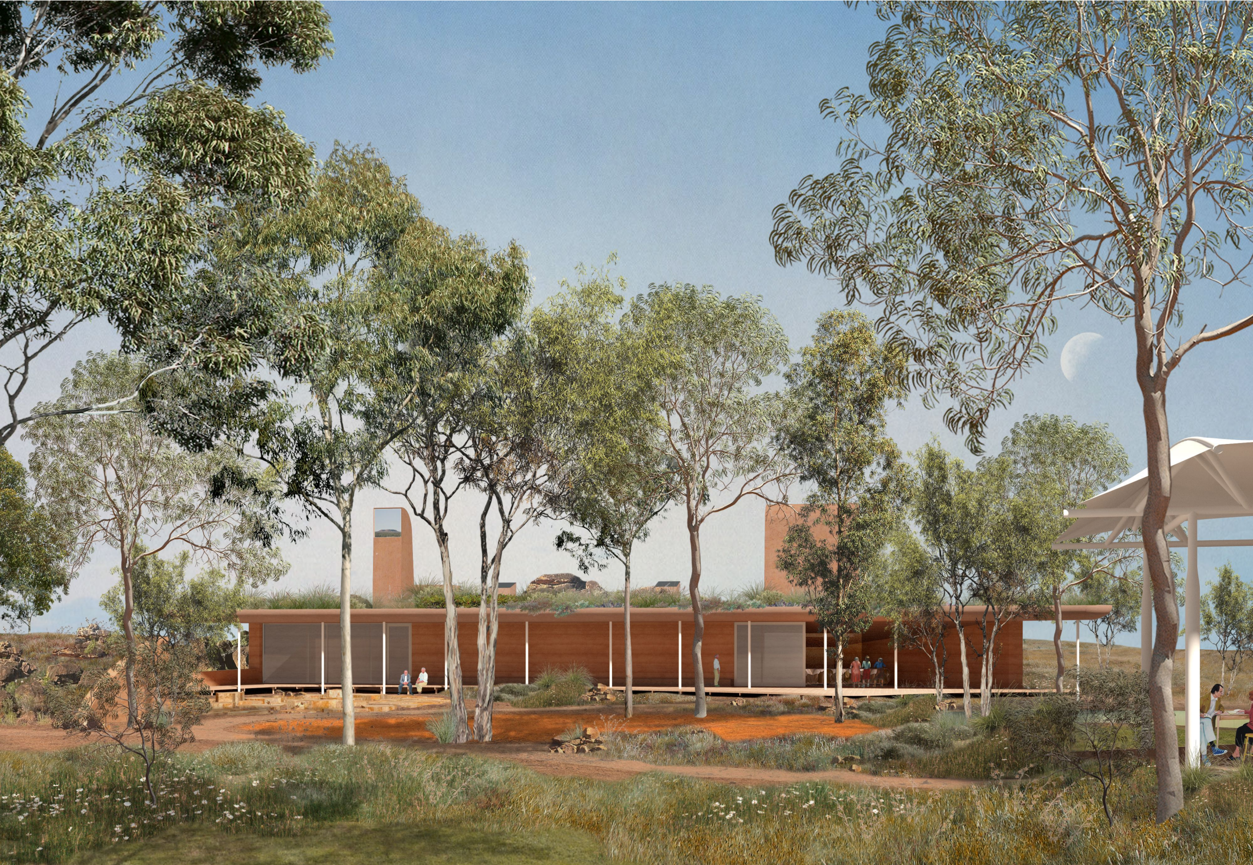
REN - Render Earth render system, using local materials
